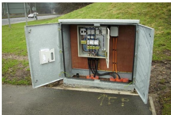
Typical installation Outgoing Impact Detector Cables
